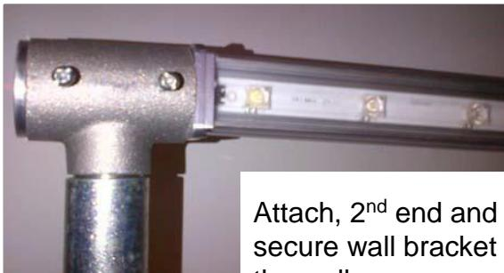
Attach, 2<sup>nd</sup> end and secure wall bracket to the wall.
